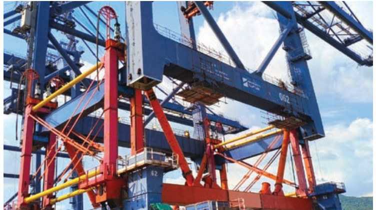
Quay crane heightening at YANTIAN.
