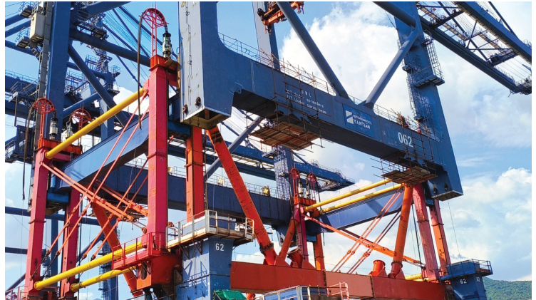
Quay crane heightening at YANTIAN.
