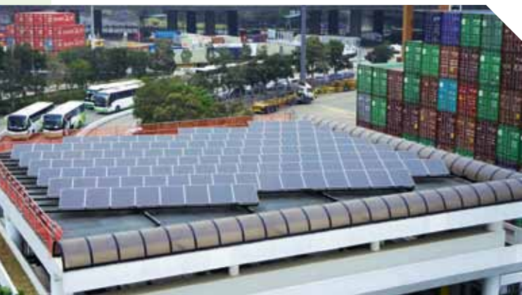
Solar panels power the emergency gatehouse at HIT
