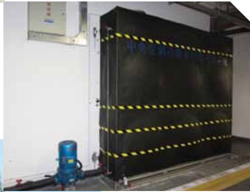
Reusing condensed water from the air-conditioning system, implemented thanks to suggestions submitted by staff
